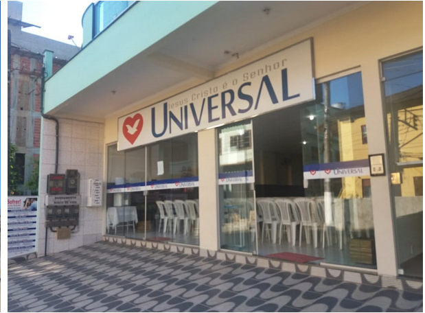
(b) Evangelical church façade
